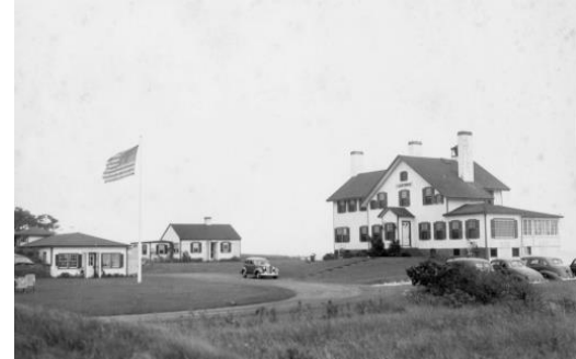
The beginning of Lighthouse Inn 1938
