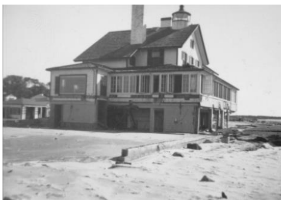
September 15, 1944 The new dining room was swept away by a hurricane. The foundation was all that remained.
