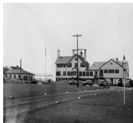
June, 1945 A new dining room and kitchen were constructed on a steel frame with walls designed to break away in the event of hurricane.
