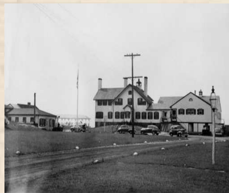
June, 1945 A new dining room and kitchen were constructed on a steel frame with walls designed to break-away in the event of hurricane.
