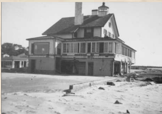
September 15, 1944 The new dining room was swept away by a hurricane. The foundation was all that remained
